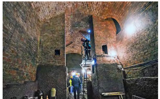
Paddington - Level 3 looking from the Lomax Chamber towards the Boote Chamber
